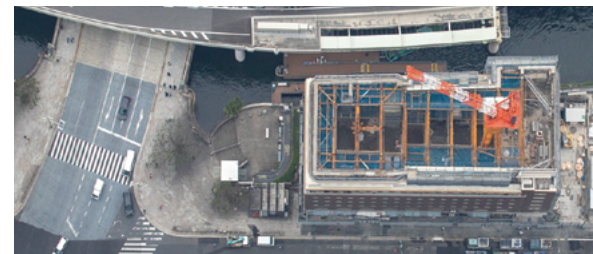
The historical building under renovation, with only the exterior walls remaining
