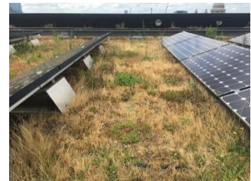
The west side of the roof in June prior to being irrigated. The grass is tinder dry and even the sedum is starting to wither.
