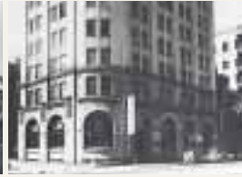
The Kitahama Nomura Building
