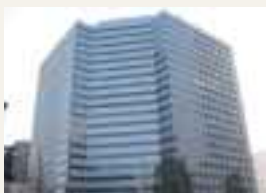
The Otemachi Head Office Building
